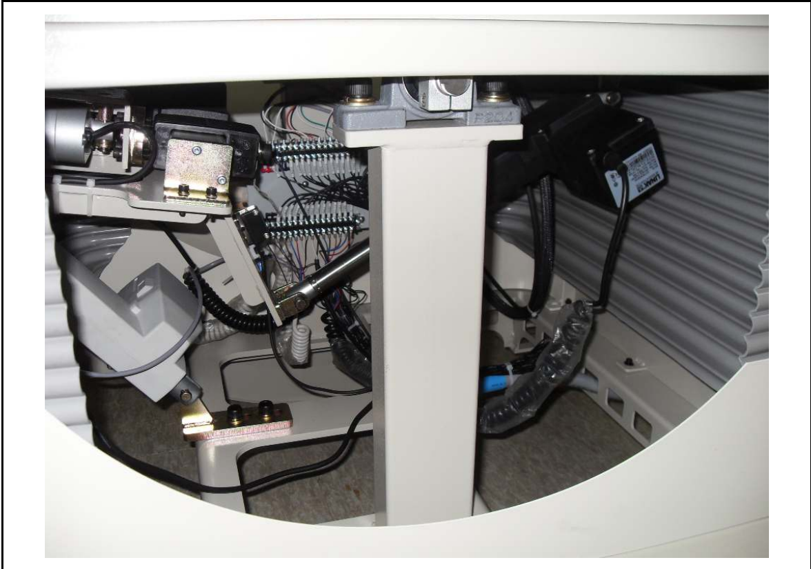
Fig. 5 : Inside view (DC motors)
